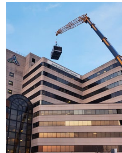
Cooling Tower Replacement NASHVILLE
